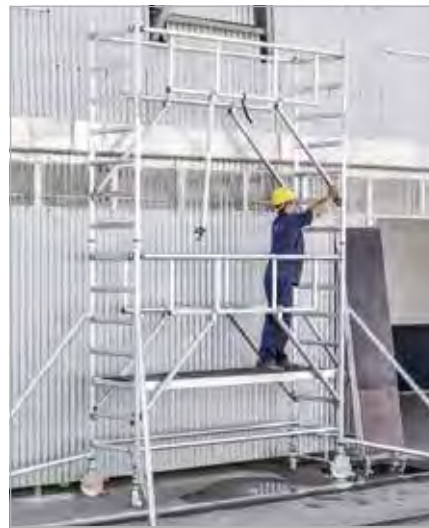
2. Attach guardrail to rungs
