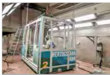
Preparation for applying anti-corrosion protection
