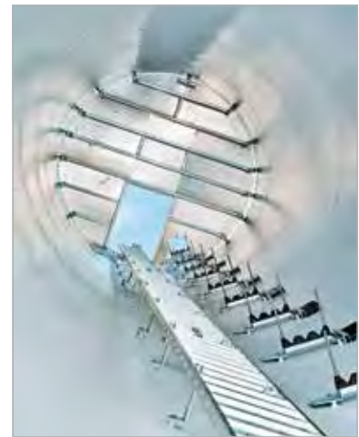
Access ladder and platform
