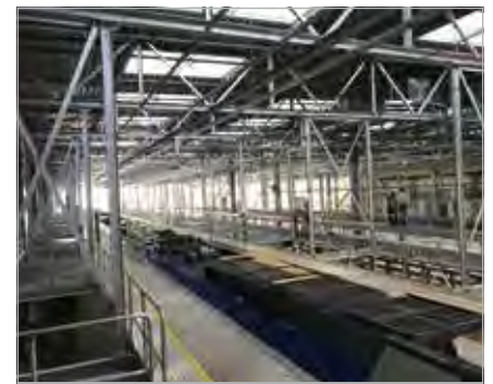
Roof work scaffolding with approx. 600m length including material lifts, cranes and PPE
