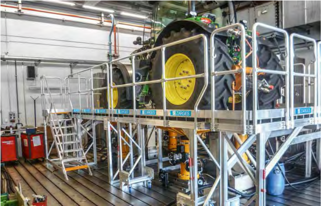
Working platform with step access.
