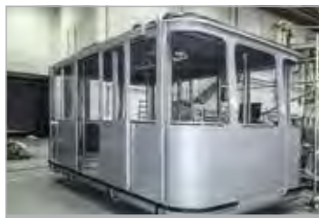
Painted car shortly before completion of work
