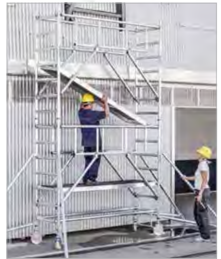
3. Hook in platform from a secured position
